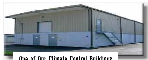
One of Our Climate Control Buildings
